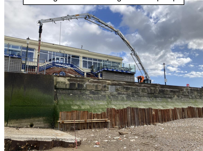
Pouring of concrete using concrete pump
