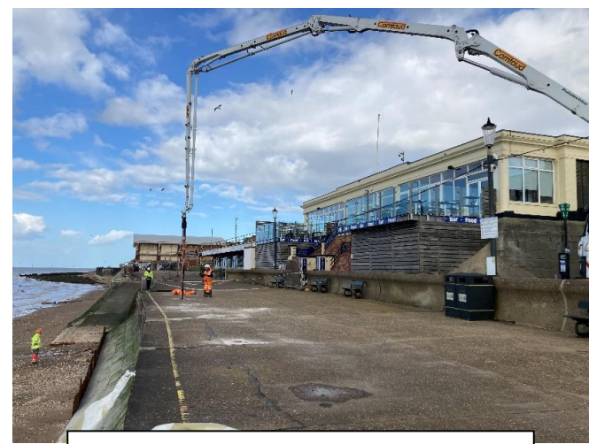
Pouring of concrete using concrete pump
