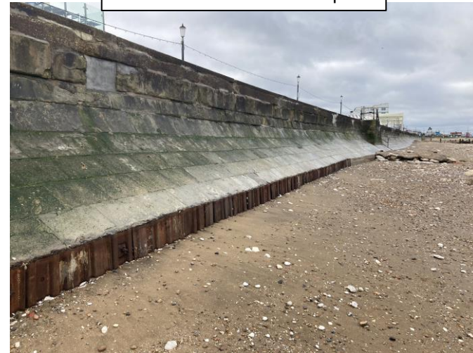
Installation of steel trench piles
