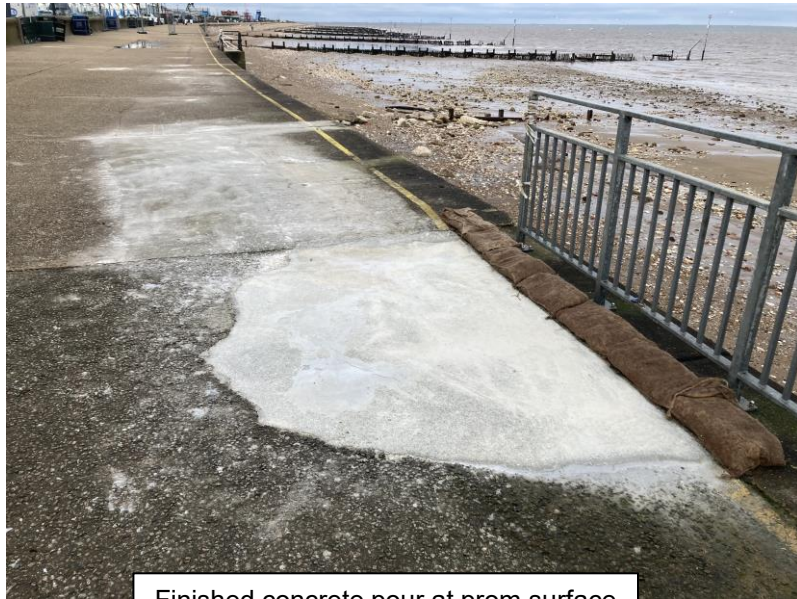
Finished concrete pour at prom surface
