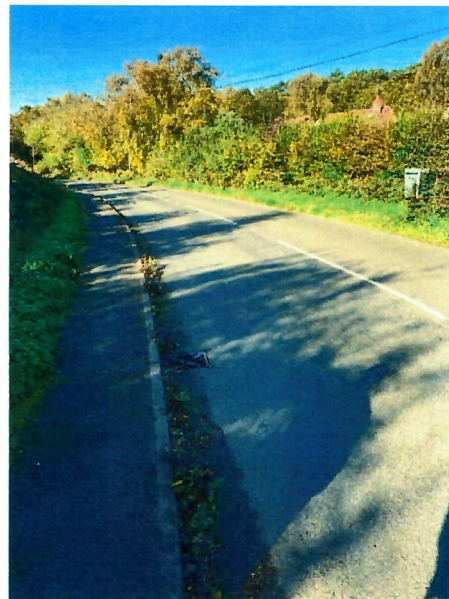
Figure 2.2 | Surfaced Footway on South Side of Beach Road
